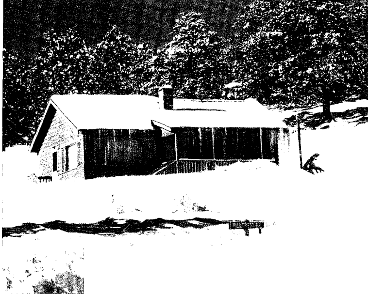
Fig. 3. East face of a cabin (12/30/06). The South Eave Effect is starting to develop on the left of the roof, and the piled up snow on the overhanging north eave at the right is a demonstration of the North Eave Effect.
