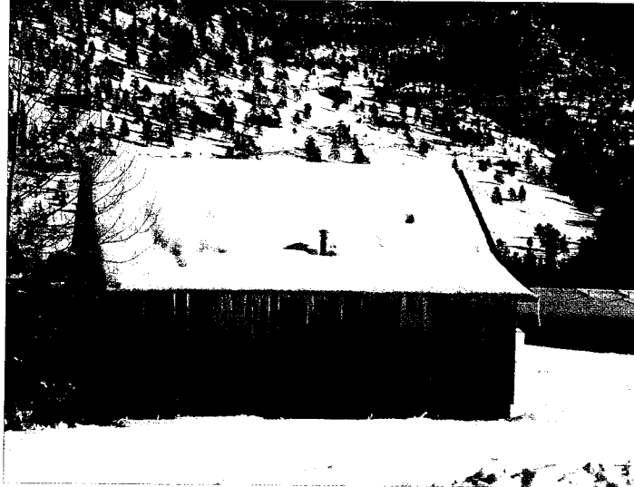
Fig. 2. West face of a cabin (12/31/06). The South Eave Effect is seen clearly on the south edge of the roof at the right.
