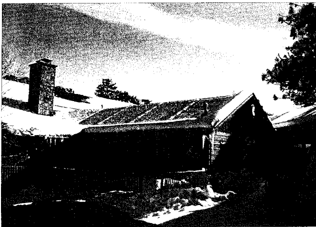
Fig. 5. Looking southeast at the north roof of a lodge building. This roof appears to be a superhighway for the escape of heat from the interior of the building. The large thickness of snow on the lower edge of the roof and on the right (west) edge are examples of the North Eave Effect (12/31/06).
